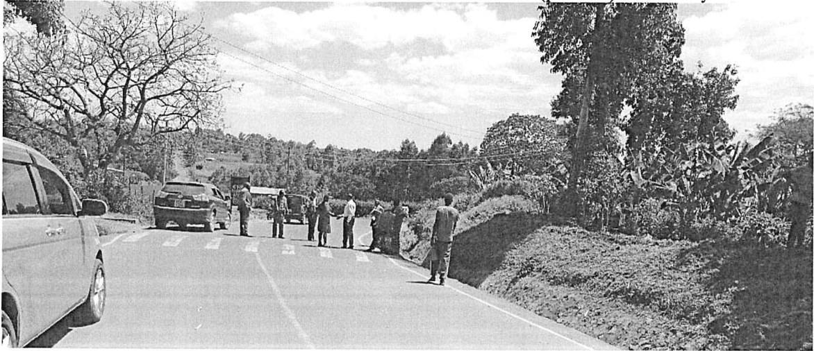
The Upgraded Riziki to DC Road(C33), towards Slaughter House
