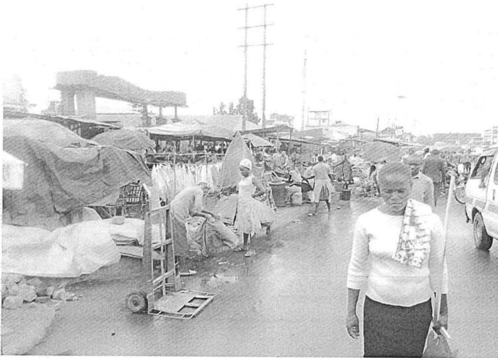
A section of the road encroached by traders and transporters
