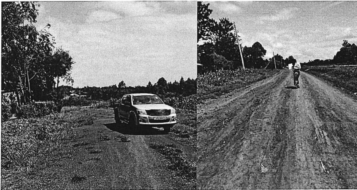
A section of Lumoro-Namirembe Dispensary road
