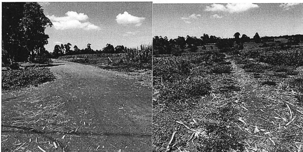
Sections of Mulukhu Road
