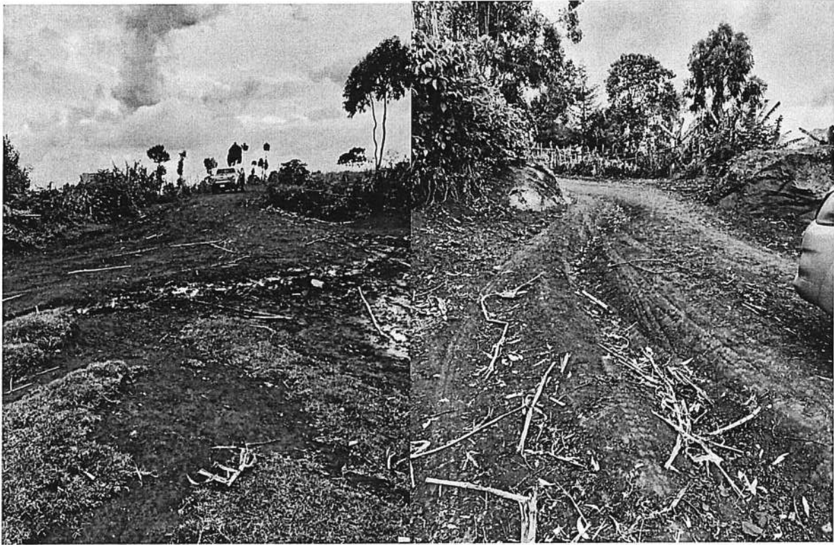
A section of Kamuneru Main - Kimakina Road
