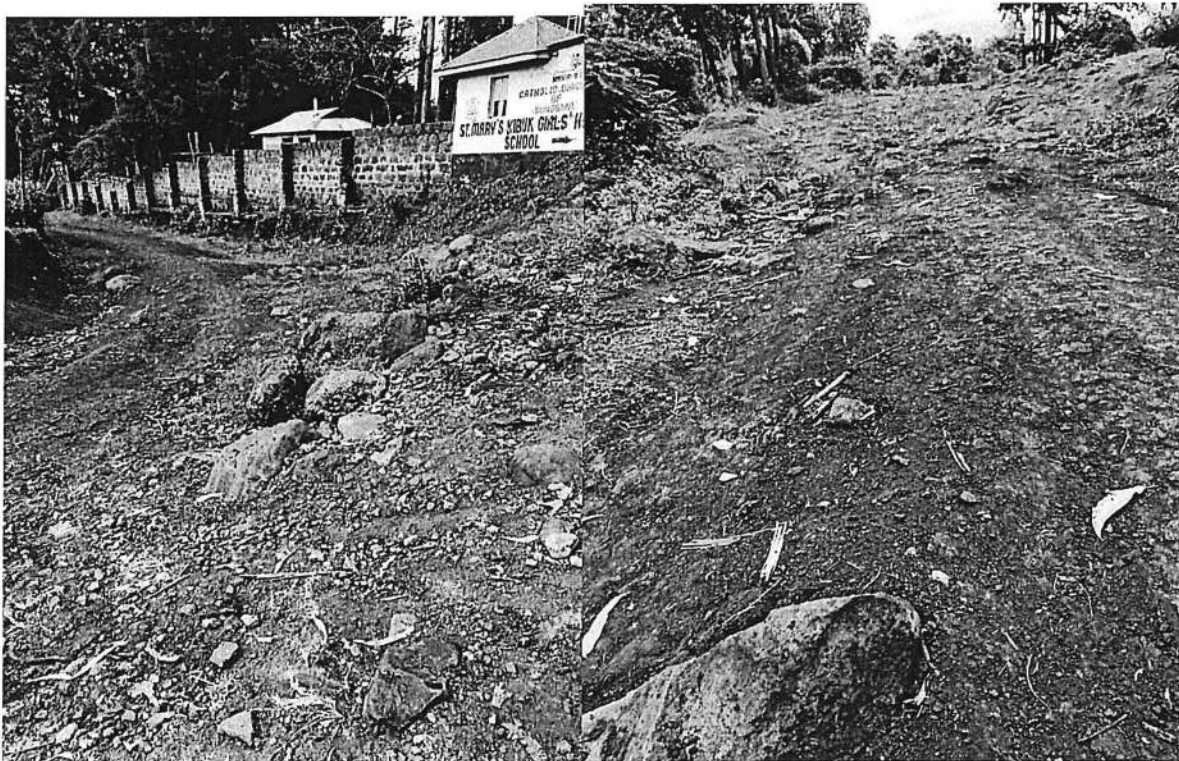
A section of Kibuk-Chepkui road
