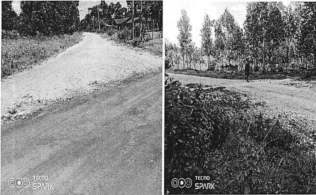
Section of Sichei cattle dip-Chwele River Road
