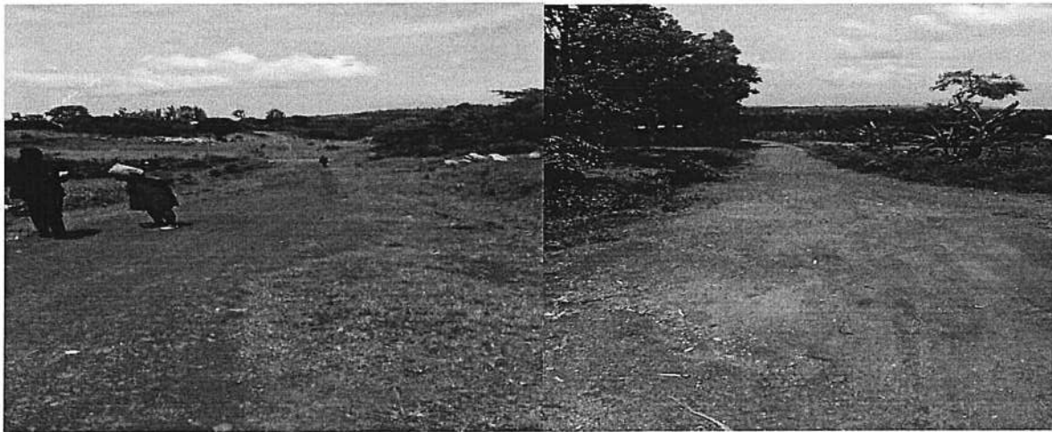
A section of Bukiyabi-Kaburweti-Namutokholo-Lwakhakha Border Road
