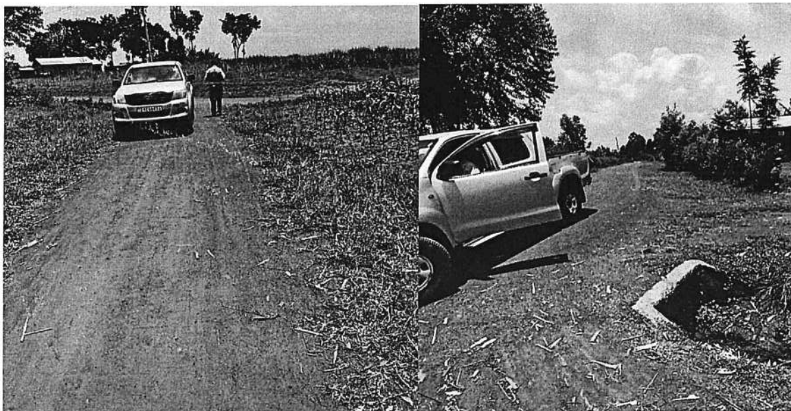
A section of Elima -Fuchani Road
