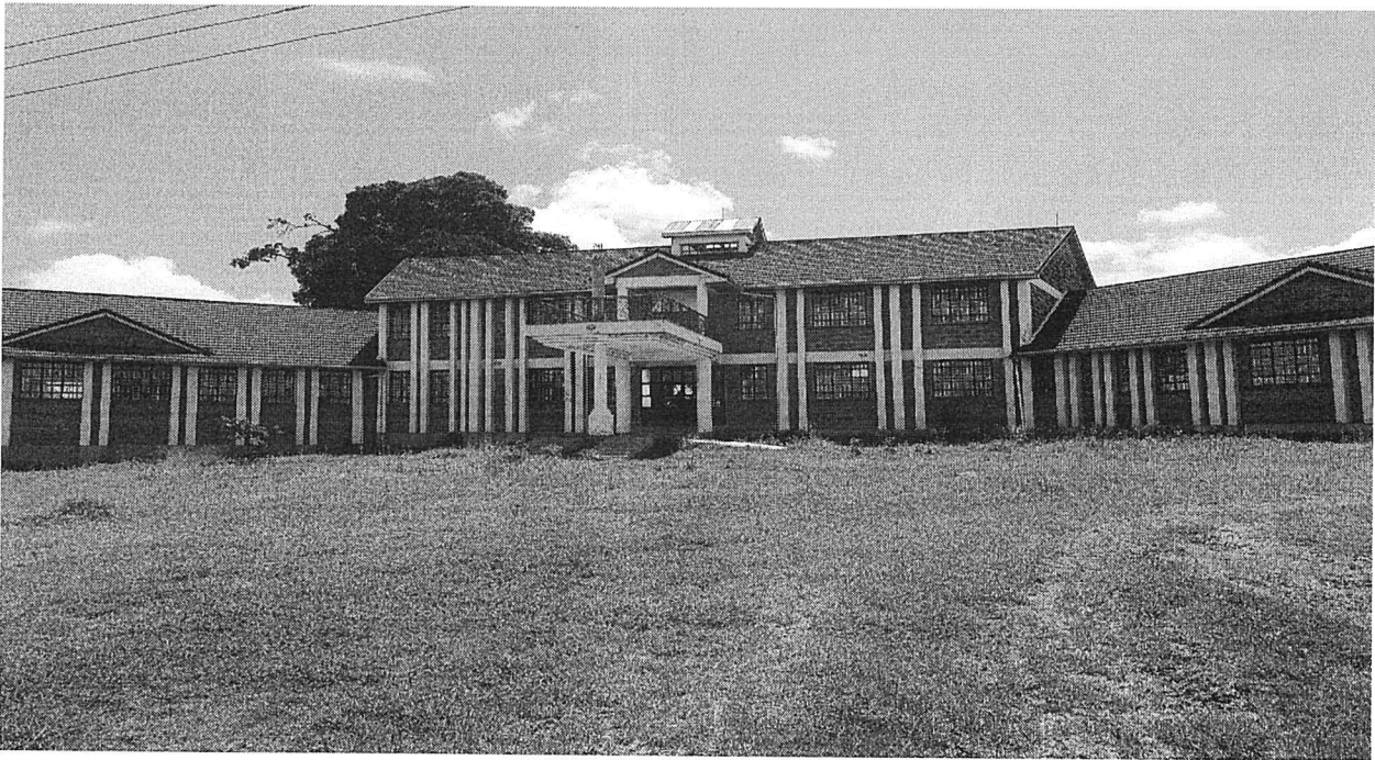
Figure 2: Complete Administration Block
