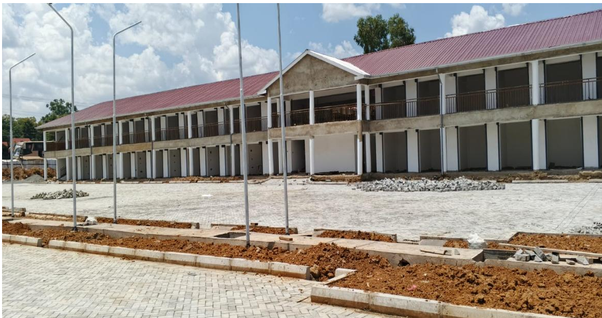
Figure 4: Modern bus park in Kanduyi
