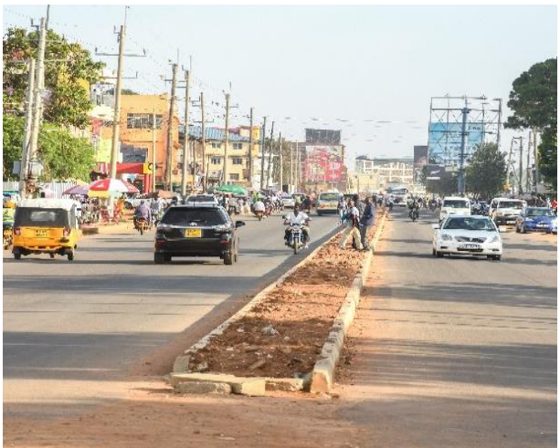
Dual carriageway road in Bungoma Town
