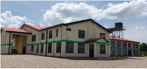
Dairy Processing Plant Structures at Webuye
