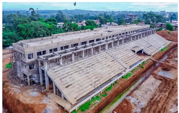
Modernization of Masinde Muliro Stadium
