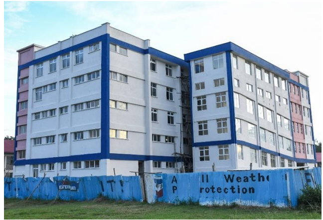
Maternity wing at Bungoma Referral Hospital
